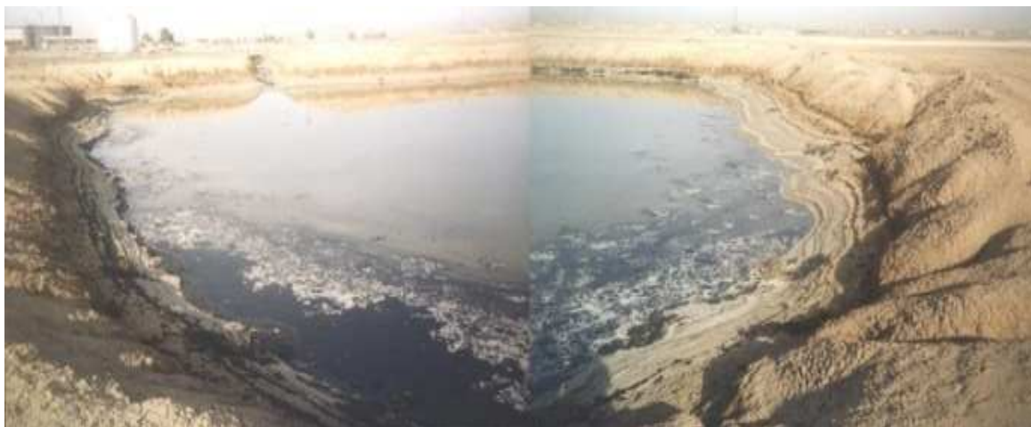
Fig.3. Waste Water Pit of Oil - Water Separator Pound Offsite The Desalinization Plant
