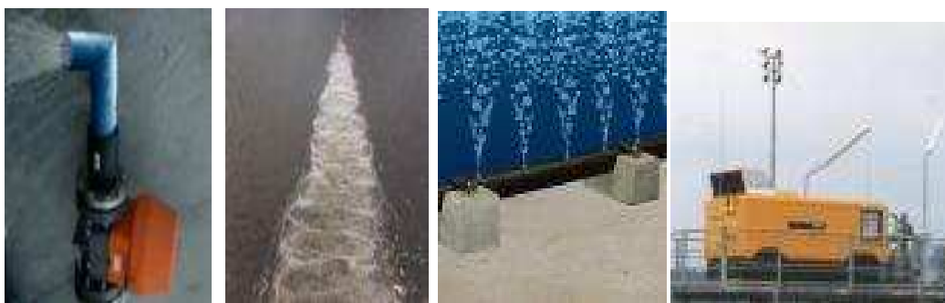
Figure 3- from the right 1 - the compressor station, 2 - pipe with special nozzles incorporated and anchor blocks, 3 - level generated by bubble curtains to the surface, 4 - the discharge valves on end of the nozzle tube.
