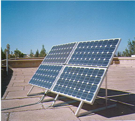
**Figure 2:** Photovoltaic panels SP75 installed at the Faculty of Science of Oujda.
