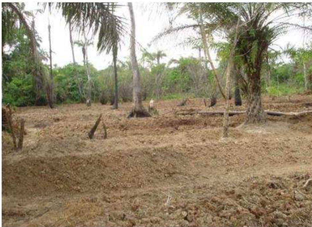
Fig 3: Windrows constructed at site II
