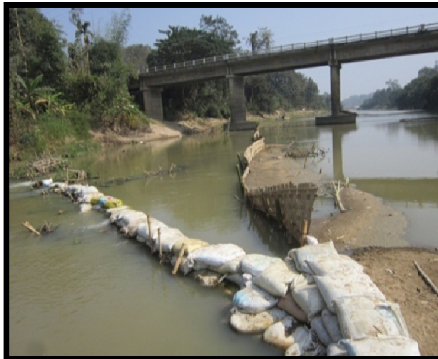
Plate 2: Obstruction in natural flow of the Muhuri River to store water for the purpose of drinking water supply near Muhuripur
