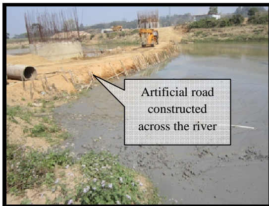
Plate 4: Sediments are deposited in the downstream section of the constructional site due to the construction of artificial road across the river
