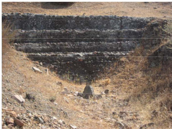
Figure 1: Staggered cyclopean concrete wall of the Roman cistern of Cerro de La Coja.
