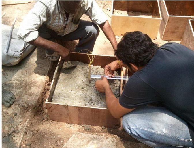
**Fig.1 Form work and placing of Thermocouple**
