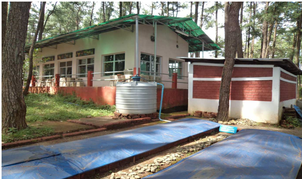
Fig 6- Underground tanks to store rain water
