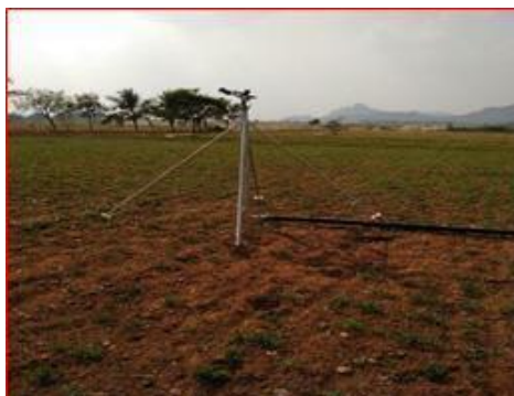
Figure 2. Installation of raingun in field
